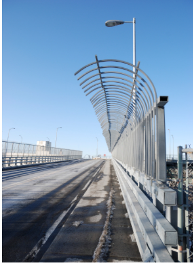
The security barrier on the Jacques-Cartier Bridge, in Montréal, was installed to prevent suicides.
