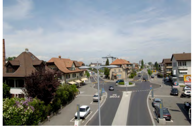
Figure 2 The through road/main street intervention: a public road for everyone
